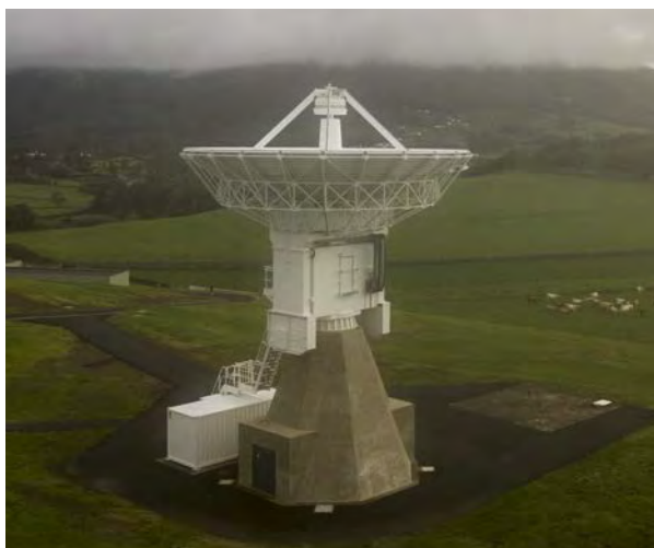
Fig. 4: Santa Maria 13.2 m station from a drone.
