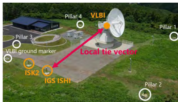
Fig. 1: Panoramic view of the Ishioka geodetic station. Four pillars and a VLBI ground marker are arranged around the VLBI telescope. The IGS station ISHI is installed about 40 m away from the VLBI telescope. ISK2 is also installed as an auxiliary for ISHI.
