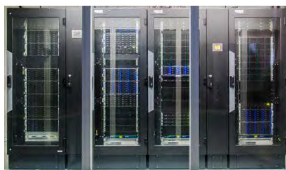
Fig. 1: New HPC cluster at MPIfR seen through a glass wall.
