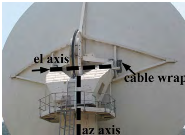
Fig. 6: HartRAO 15 m az-el mount – rotation axes and on-axis prism mounting point at west end of elevation shaft (arrow on left). The east end of the elevation shaft is obscured by the cable wrap (arrow on right).
