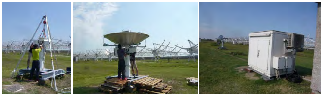
Fig. 2: Installation of transportable VLBI station at Medicina. The transportable 2.4 m antenna consists of separate assemblies for the dish and Az/El drive system. Three persons are sufficient to assemble the system in two days of work (Left and Center). A small air-conditioned box, located 30 m from the antenna, contains antenna control system(right).
