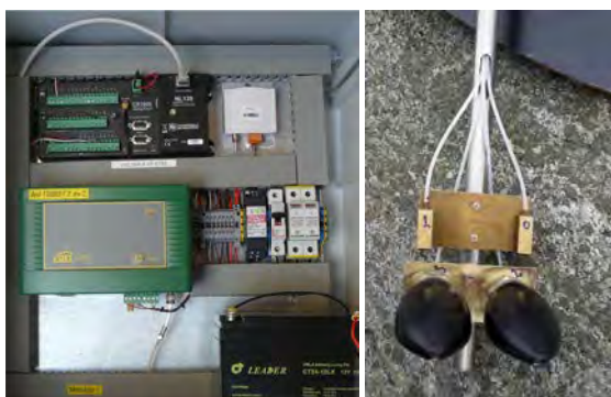
Fig. 3: The pneumatic sensors, Ott CS471 of USGS type, have a compressor (green unit, left) located in the measurement hut. Each compressor is connected to a nozzle (right) via a plastic pipe. Two nozzles are used at the bottom of the well, and one nozzle is located close to the bottom outside of the well. The original black nozzles corroded rapidly in the salty water and were replaced by the ones located just above (manufactured in copper) in October 2016 (see also Fig. 5).
