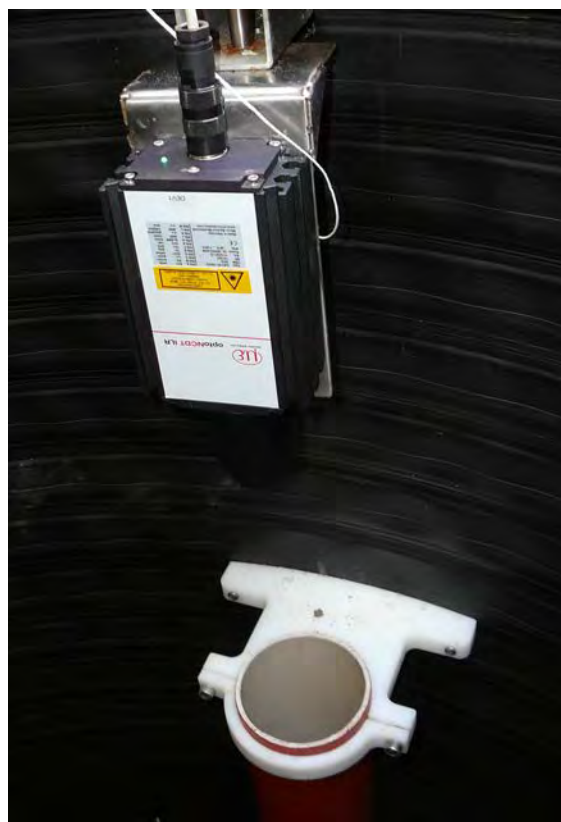
Fig. 4: The laser sensor is mounted on the inside wall of the well. A reflecting target is floating on the sea surface inside the pipe.
