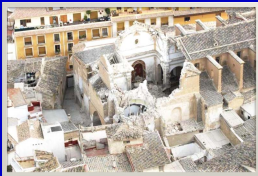
Total collapse in the Santiago Chapel in Lorca caused by the May 11, 2011 5.1 Mw Lorca Earthquake.
